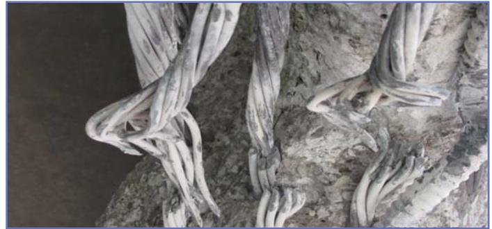
Collision-damaged strands on one of the bridge girders.
