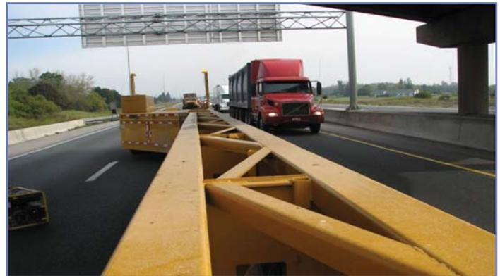
Mobile Traffic Barrier in use under the Dingman Drive Bridge.
