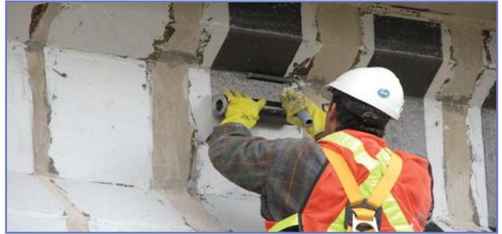
Application of CFRP strips with a roller.
